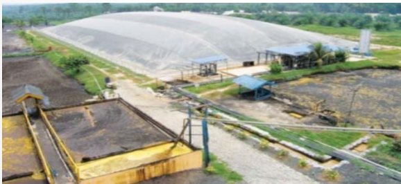
waste processors POME to be Biogas - PTPN V Riau
